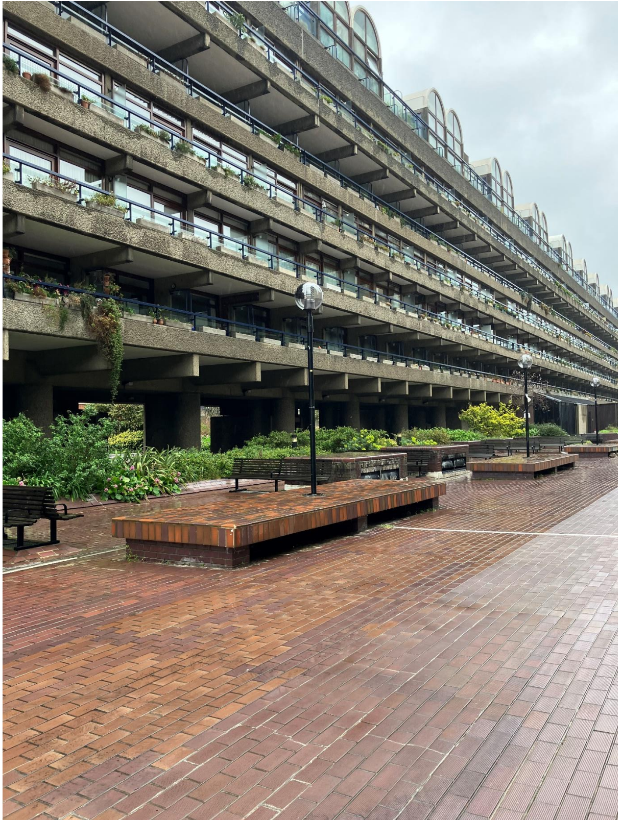
Image 6: Existing tiled benches and street furniture on the Podium, with the mismatched tiles found across the space as a result of ad-hoc works.
