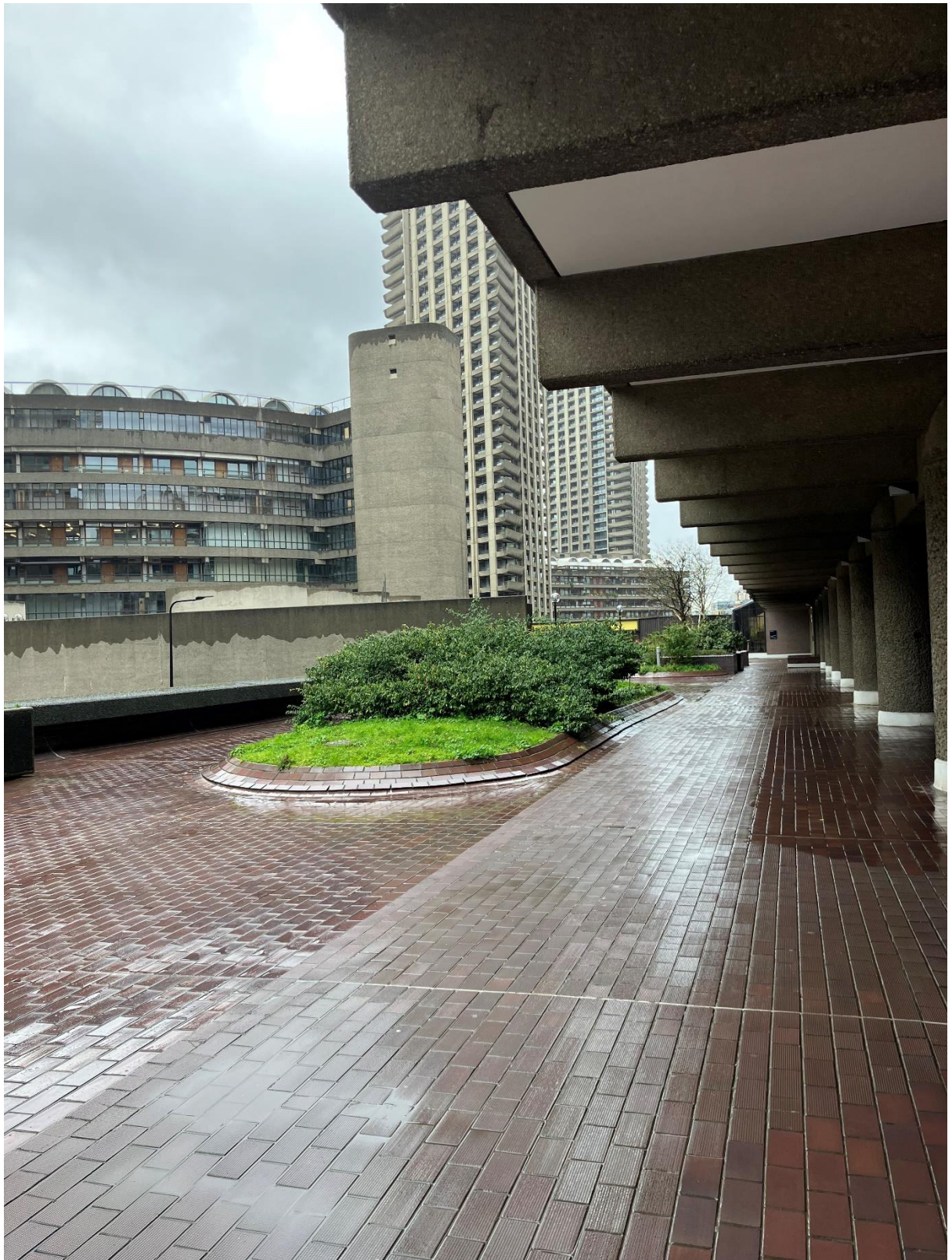
Image 2: Podium looking westward towards the existing Link Building
